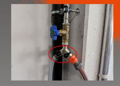
*If they are closed, you can open the blue valve until the end. An orange ring should be visible.*
