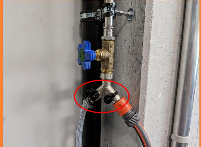
If they are closed, you can open the blue valve until the end. An orange ring should be visible.
